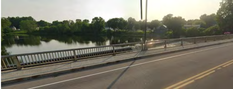
Photo 1. View of Swanton Dam from Merchant's Row Road (Google Street View)
